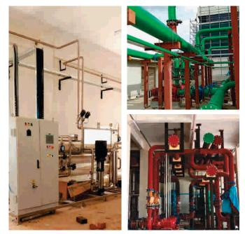
Site Location : Tumkur, Bengaluru. Scope of Work : Supply & Fabrication, Erection of Utility Piping , Chiller Installation and Commissioning jobs, Water Purifier System, Technical Area Piping in Pharma Plant
